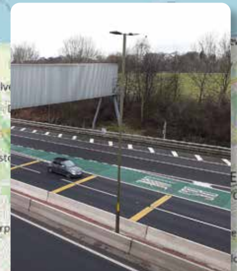
Refreshed road markings
